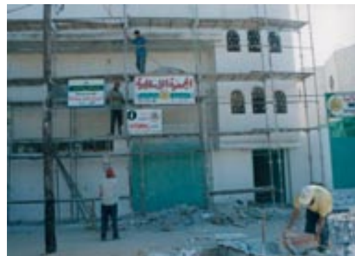
Construction work on the Orphan Centre in Jabalia, supported by Interpal
